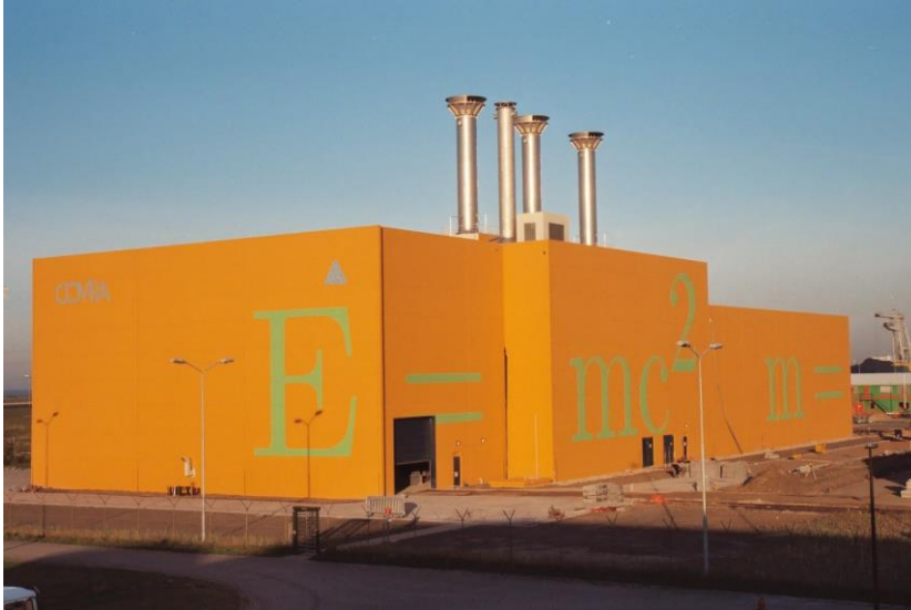
Figure 5. HABOG shortly before completion
