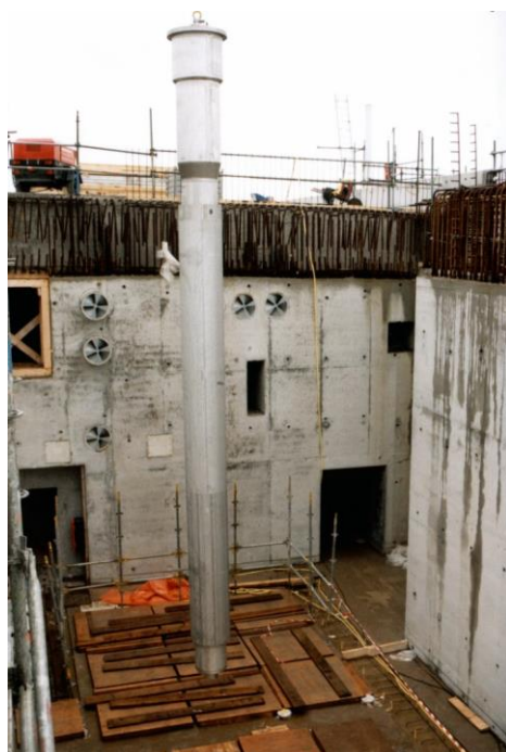
Figure 4. Emplacement of the wells during construction
