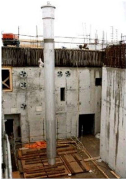
Figure A.4. Emplacement of the wells during construction
