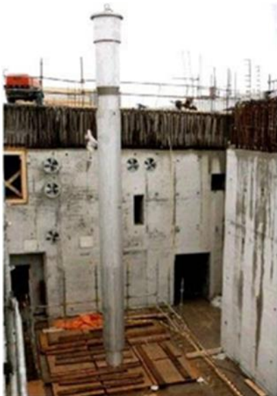
Figure A.4 Emplacement of wells during construction
